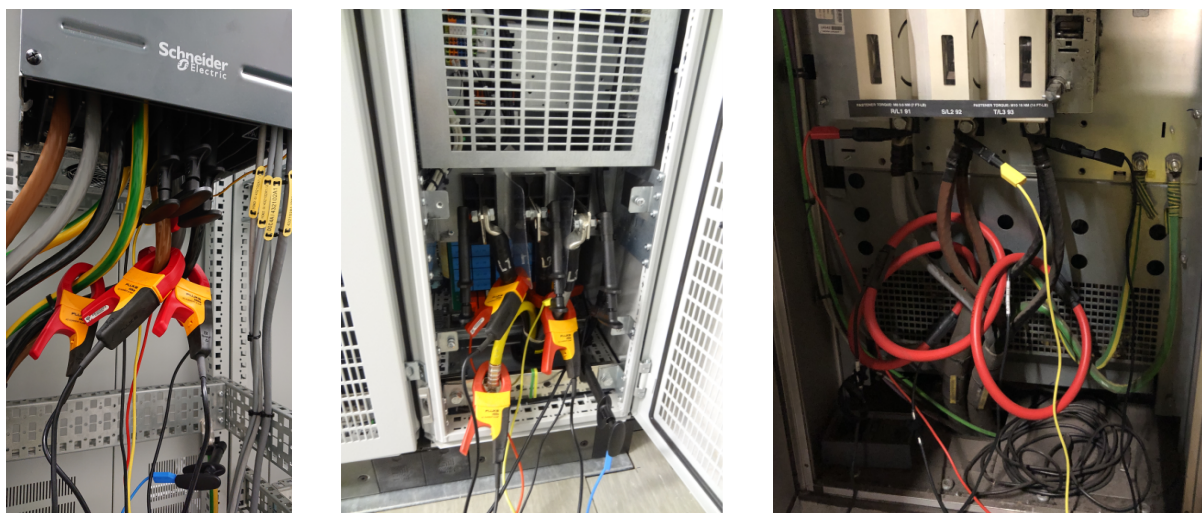
Figure 6: Measuring at the VFD-side (the preferred option)
