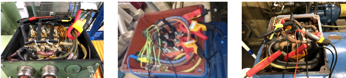
Figure 5: Measuring at the terminal box (not the preferred option)
